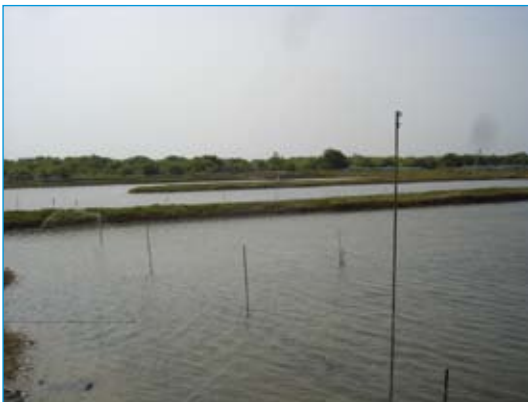
Reservoir with baffles
