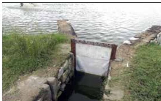
GAQP-Well maintained sluice gate for efficient water regulation in biosecured L. vannamei farms
