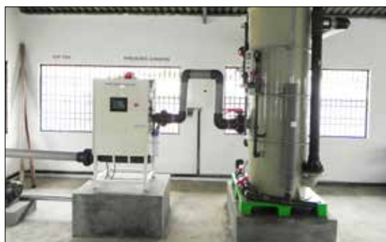
GAqP - Refrigeration and Hypochlorus Generator in a biosecured L. vannamei hatchery
