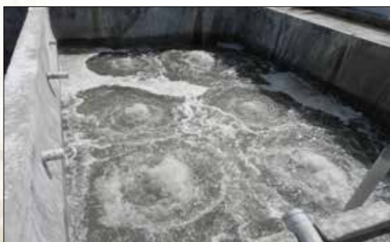
GAqP - Aeration in ETS of biosecured L. vannamei hatcheries
