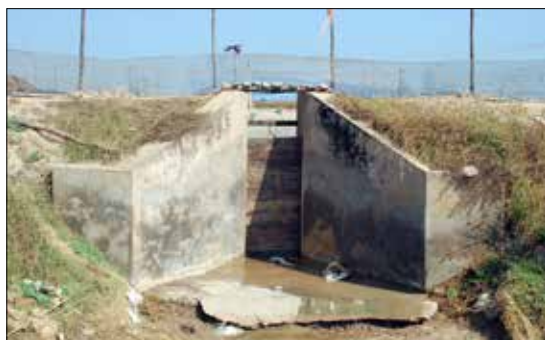
GAQP-Well maintained sluice gate for efficient water regulation in biosecured L. vannamei farms
