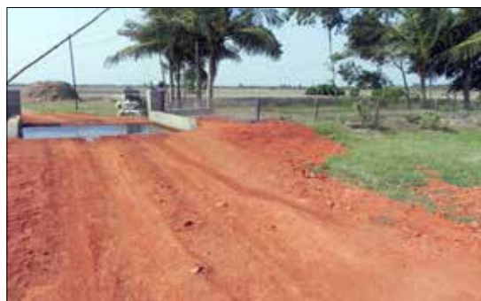
Farm fencing and tyre wash with barrier at main gate of biosecured L. vannamei farms
