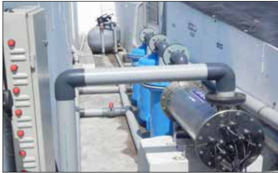
Water treatment and filtration systems in biosecured L. vannamei hatcheries
