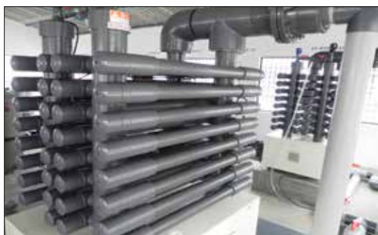
GAqP - Refrigeration and Hypochlorus Generator in a biosecured L. vannamei hatchery
