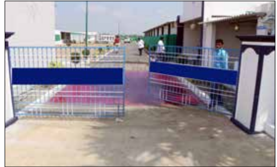
Biosecurity in hatchery-Compound wall and tyre wash
