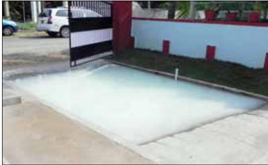
Biosecurity in hatchery-Compound wall and tyre wash
