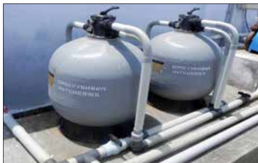
Water treatment and Filtration systems in biosecured hatchery
