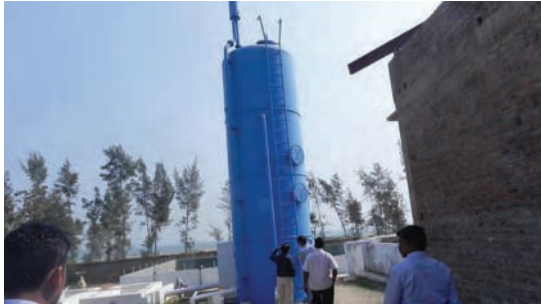
Biosecurity-Sand filter
