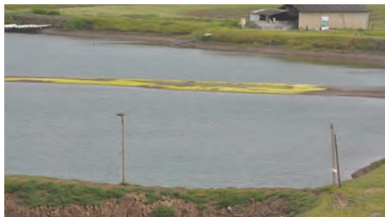
ETS for wastewater treatment
