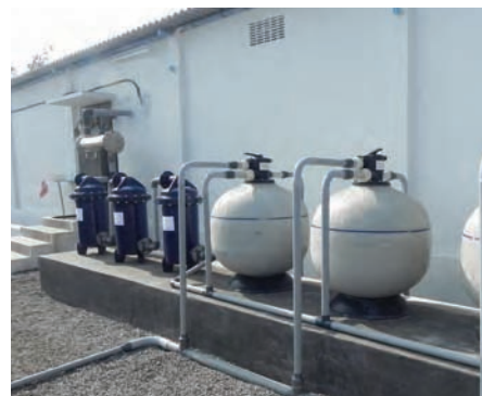
Water treatment and Filtration systems in biosecured hatchery
