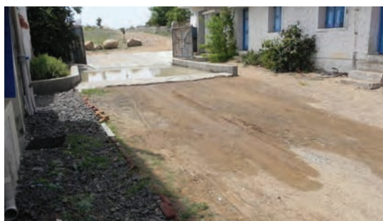
Biosecurity in hatchery-Compound wall and tyre wash
